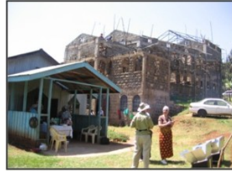
View of existing church building (on left) beside new building
