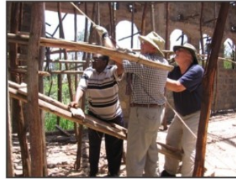
Helping to raise roof trusses
